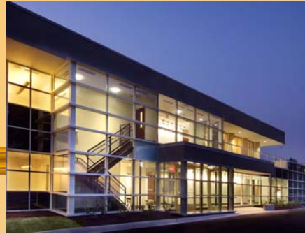
ASHRAE Headquarters - Atlanta, GA
