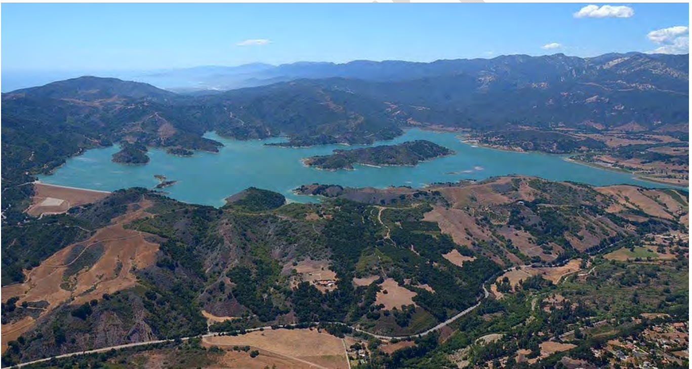
FIGURE 4-2 LAKE CASITAS AND CASITAS DAM
