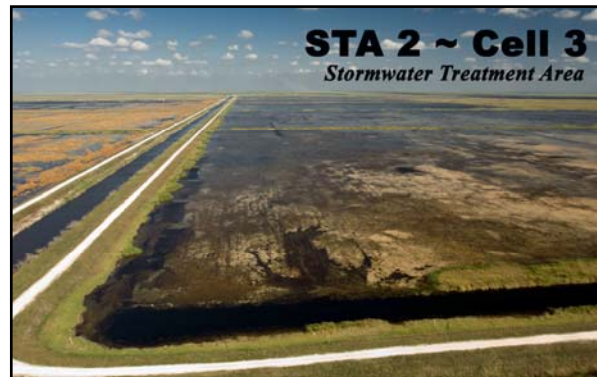
Stormwater Treatment Areas (STA) are manmade marshes designed to remove phosphorus and other pollutants from the water column. The Essentials document that almost double the acreage proposed in CERP will be needed for STAs in order to treat all of the water.
