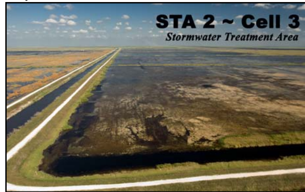
Stormwater Treatment Areas (STA) are manmade marshes designed to remove phosphorus and other pollutants from the water column. The Essentials document that almost double the acreage proposed in CERP will be needed for STAs in order to treat all of the water.
