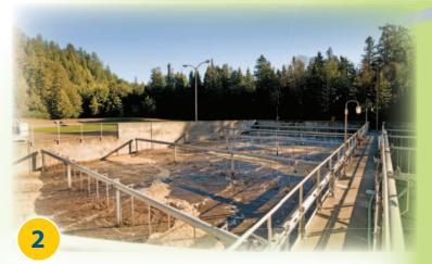
Aeration Basins The wastewater undergoes biological treatment in the aeration basins. Air is injected into the wastewater to promote the growth of microorganisms that feed on organic materials in the sewage.
